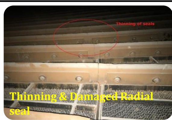
APH Damaged Seal replaced with new one
